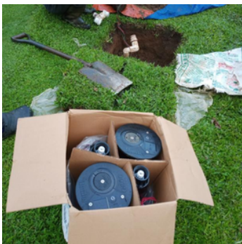
INSTALLATION OF BRAND NEW SPRINKLERS
