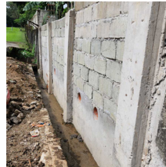
CONSTRUCTION OF PERIMETER FENCE
