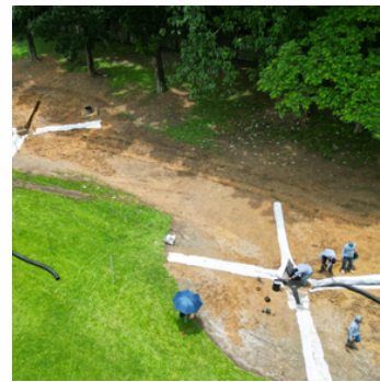
DRAINAGE IMPROVEMENT AT HOLE # 4 NORTH COURSE
