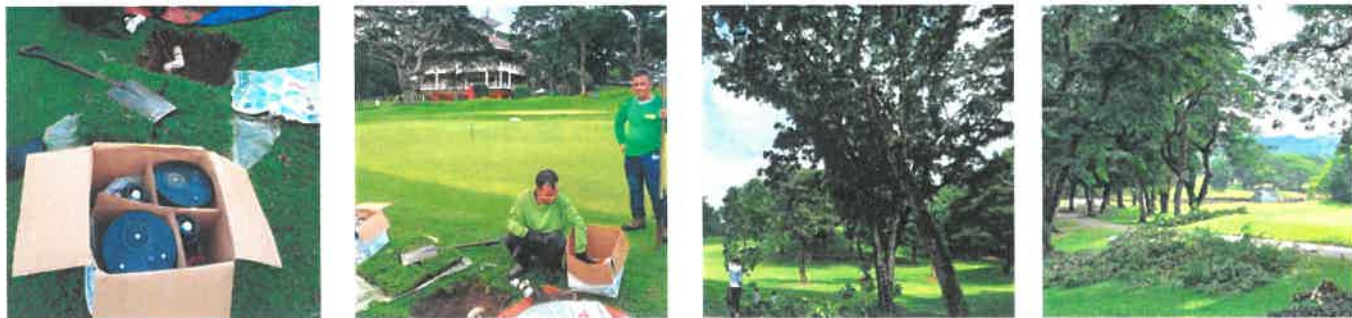
INSTALLATION OF BRAND NEW SPRINKLERS
